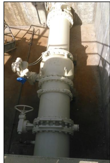
New plant Influent valve
